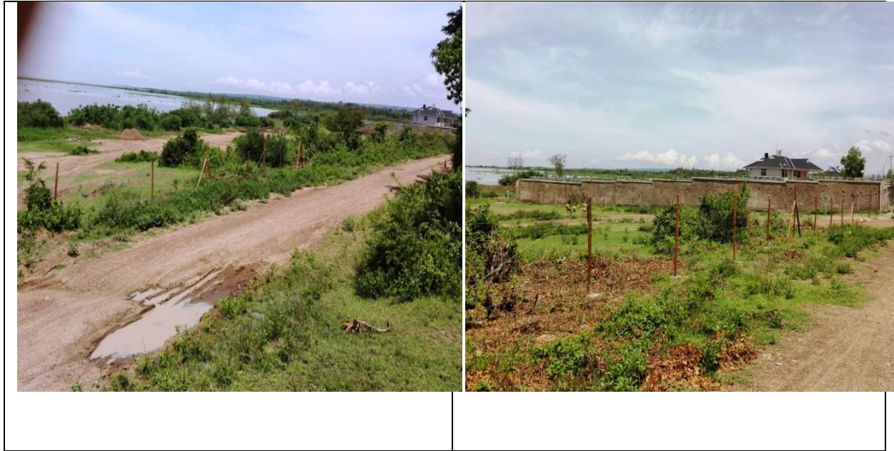
Figure 4.19: Wall fence encroaching unto the lake ( left ) and a newly fenced plot encroaching the lake ( right )
