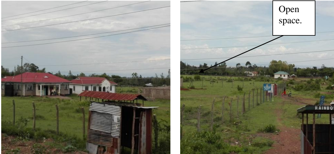
Figure 4.4: Institutional developments showing public health centre to the left and Chiefs office to the right
