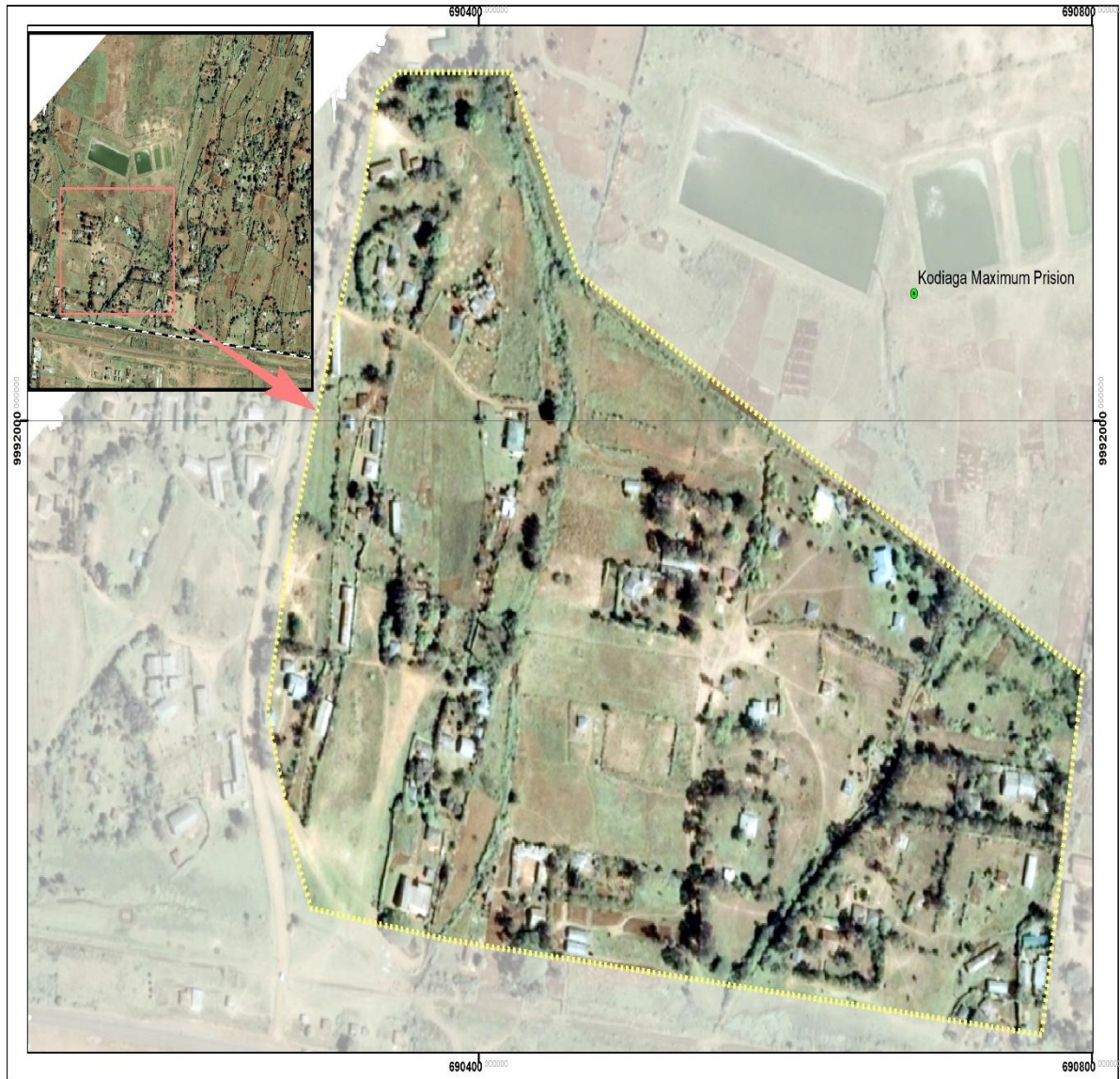
Figure 4. 16: The density of development in 2009 in a section in the study area (Source: Google Earth images redrawn by author)
