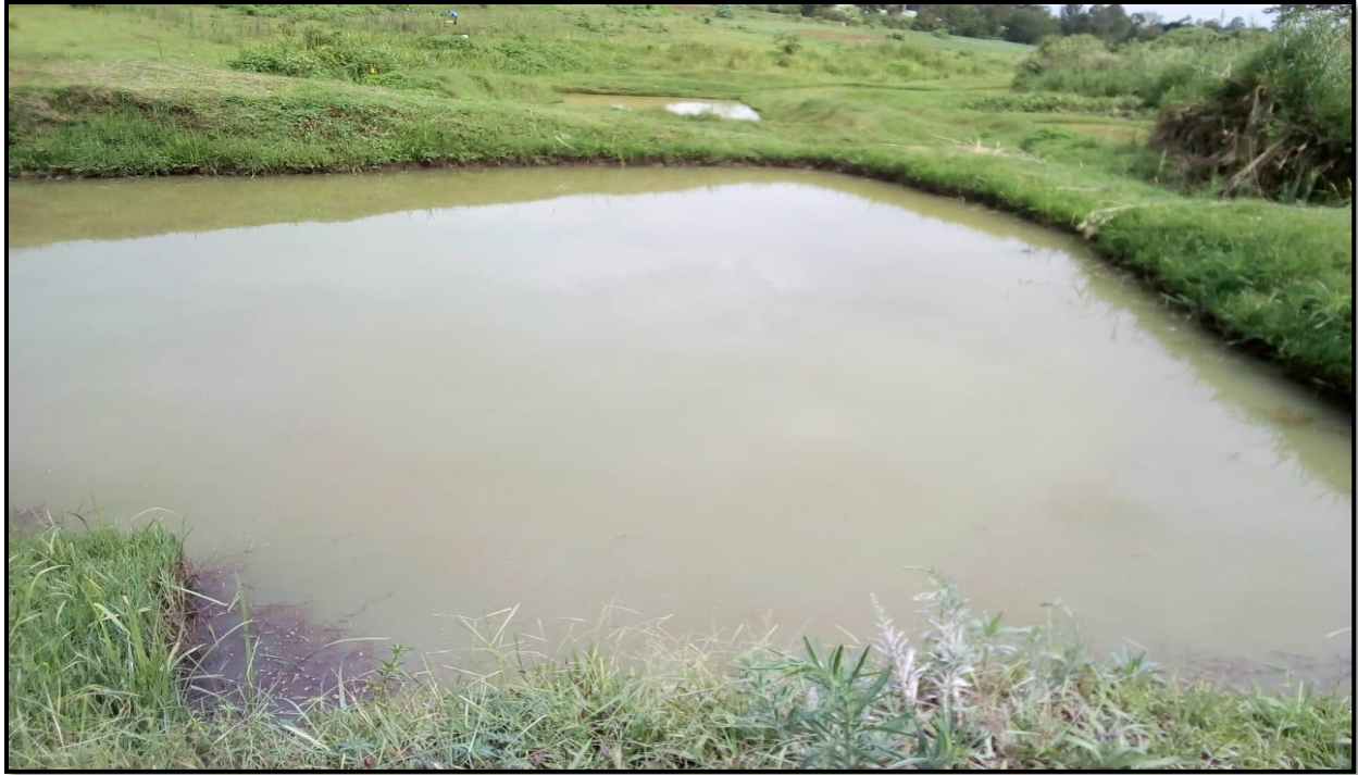
Figure 4.3 Pond funded through ESP at Ojolla, South West Kisumu Ward
