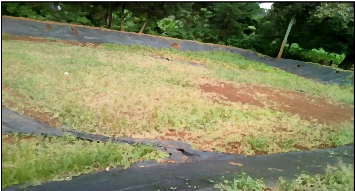
Figure 4.2 Pond within Kogony, Central Kisumu Ward not fully covered by a pond liner
