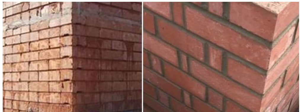
Figure 1. Modern earth blocks used in the construction of walls of houses (images taken from houses under construction in Busia Country, Kenya).
